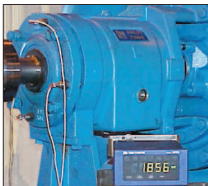
Bearing Load Measured on Test
