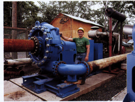
Portable diesel driven 5500 pumping gravel.
