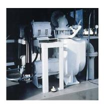
Trash Hogs are utilized in remote sewage lift stations to pump municipal waste from outlying residential areas to the local treatment plant. Here, Trash Hogs are being driven by overhead belt drives to conserve lift station space. Service will be performed by removing the rotating element to the rear as typical suction piping restricts access to the front of the pumps.
