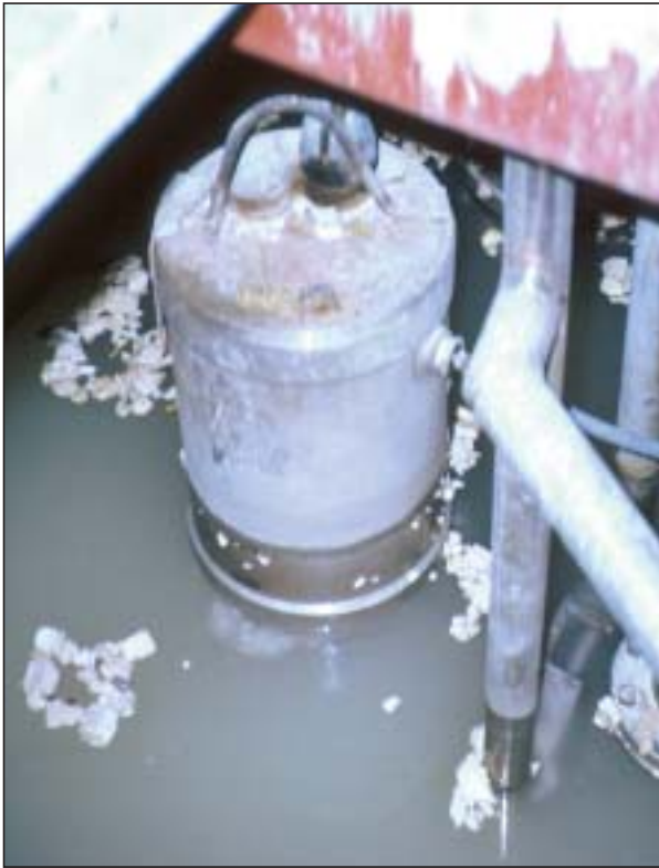
Picture 1 shows one of two Grundfos stainless steel pumps used for pumping pigment-containing channel water with a density of 1.0 - 1.4 kg/dm 3 and a maximum viscosity of 250 mPas. Both pumps are fitted with the patented shaft seal flushing system.
