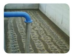
The Zenit range includes both disc-shaped and tubular membrane air diffusers.
